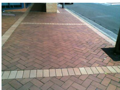
Red Brick Paving - medium-good condition
